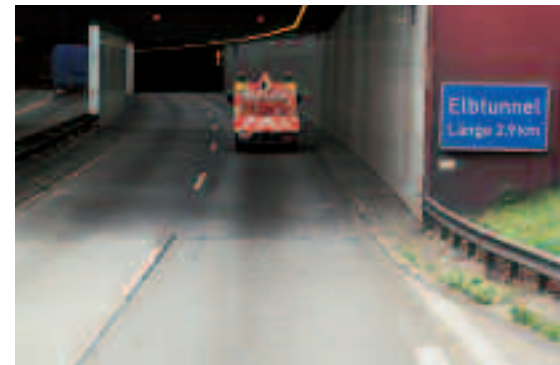
The Elb tunnel in Hamburg where the asphalt is made with Luxovit®.
